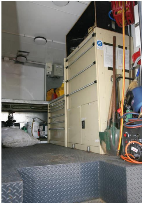
Figure 45-11: DMV's Rear Interior Metal Drawer Storage
