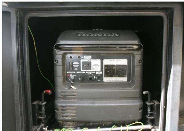
Figure 45-3: DMV's Portable Generator Compartment
