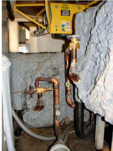
Figure 50B-9: 5080DE Aircraft Air-conditioning Unit Evaporators
