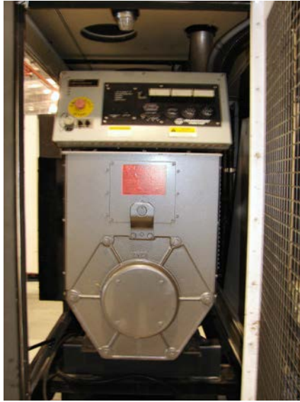
Figure 50B-11: 5080DE Aircraft Air-conditioning Unit's Motor Control Panel
