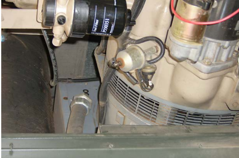
Figure 50A-7: TEC 300 AC Aircraft Air-conditioning Unit Condenser Alternator
