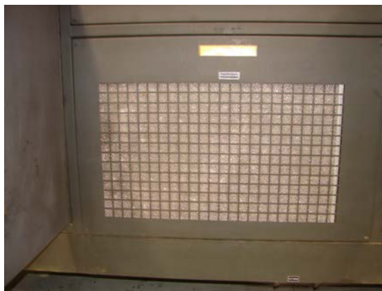
Figure 50B-2: 5080DE Aircraft Air-conditioning Unit's Filter
